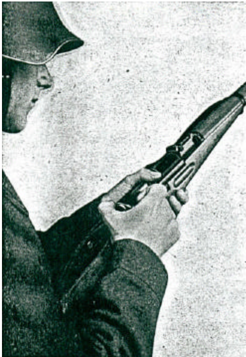
Fig.36 Removing cartridges: Opening the Bolt
