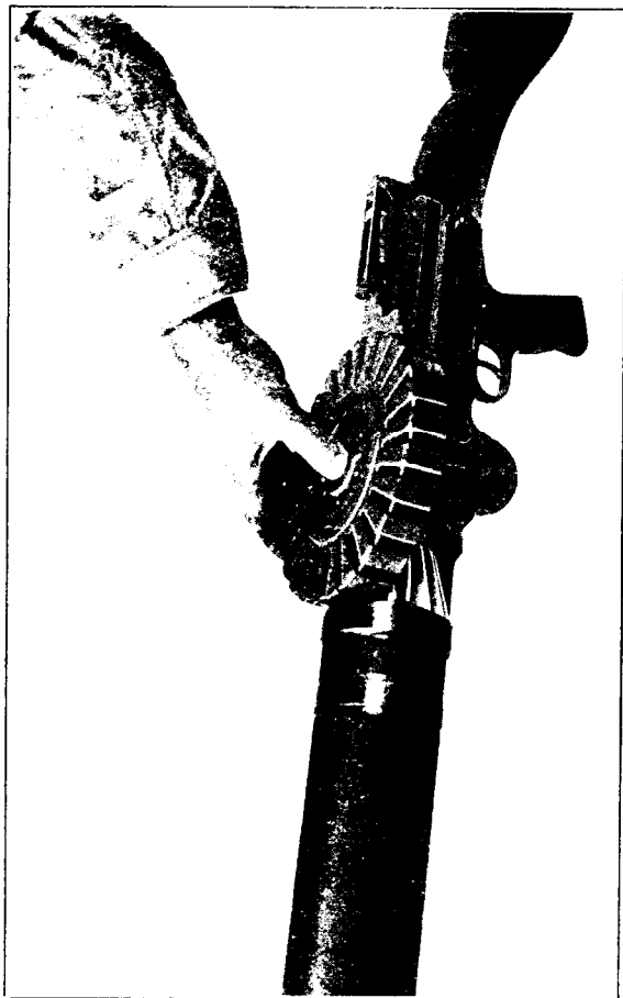
PLATE XII- VIEW SHOWING PROPER METHOD OF PLACING MAGAZINE ON MAGAZINE POST
