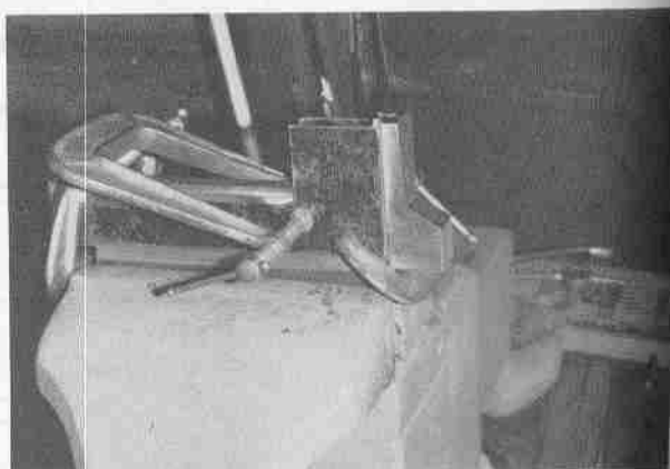
Clamped in place for welding. Note that a filler block is inserted to keep the assembly square and maintain dimensions.
